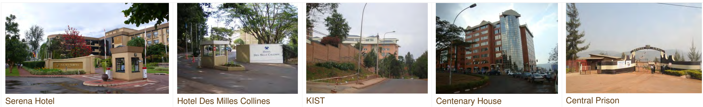
Figure 5.31: Nyarugenge CBD Landmarks - Existing Developments. Source: Surbana
