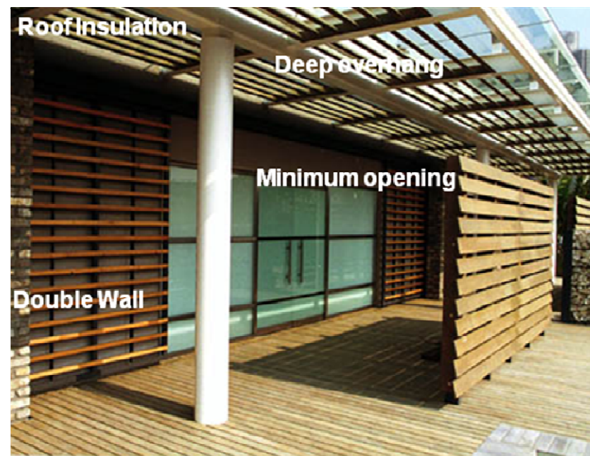
Figure A 3.6: Hong Kong Wetland Park - Use of Passive Technologies for Lighting and Ventilation. Source: Surbana
